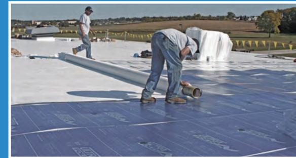
**CUSTOM PRE-FABRICATED SYSTEM** is manufactured specifically for each roofing project to ensure minimal waste and optimal fit.
