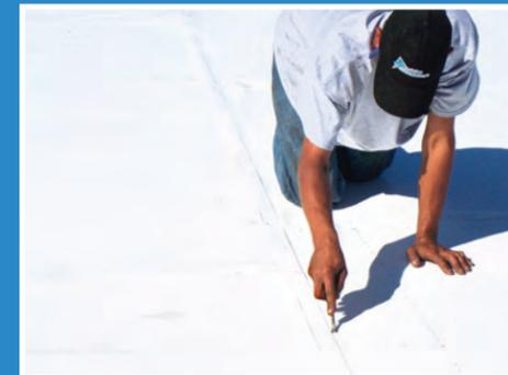
Upon completion of your roof, **WE CAREFULLY CHECK EACH SEAM.** A second inspection occurs by the manufacturer of the membrane roofing system and the comprehensive warranty goes into effect.
